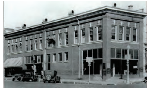
Before photo by City of Clinton
